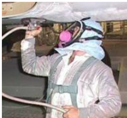
Spray Applying Sur-Prep® AP-1
